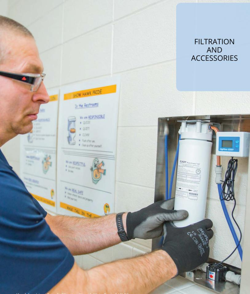
Vandal-resistant Retrofit Filtration Kit with WaterSentry<sup>®</sup> VII Filter EF1500VRBMC
